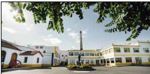
'Kendel receive further MAJOR Order from Arehucas Rum factory on Gran Canaria.'
